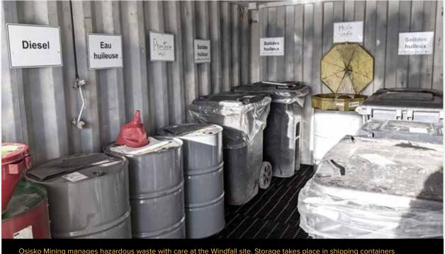
equipped with mesh floors to provide secondary containment.
