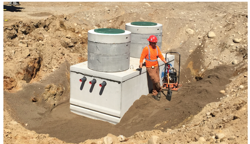
► Windfall Lake Project’s new septic field
