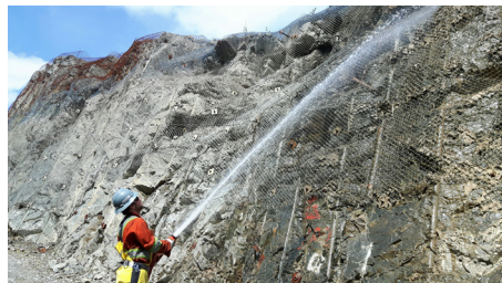
► The exploration ramp portal rehabilitation at Windfall Lake Project is complete.
