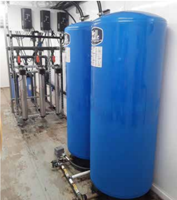
A UV lamp system facilitates the water quality management.
