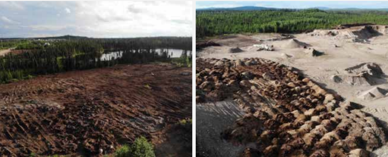
WE USED THE OVERBURDEN COLLECTED DURING THE EXPANSION OF THE LINED STOCKPILE TO BEGIN RESTORING DRILLING AREAS AND A MULTI-USERS BORROW PIT.
