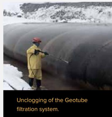
Unclogging of the Geotube filtration system.
