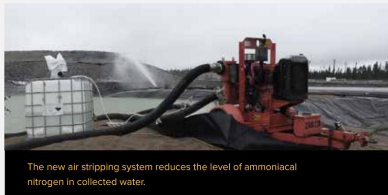
The new air stripping system reduces the level of ammoniacal nitrogen in collected water.
